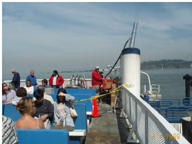
Figure 6: RAVEM system and exhaust pipe extension installed aboard Golden Gate
